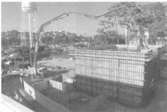
Figure 1-4 Concrete pour for a cast-in-place concrete construction
