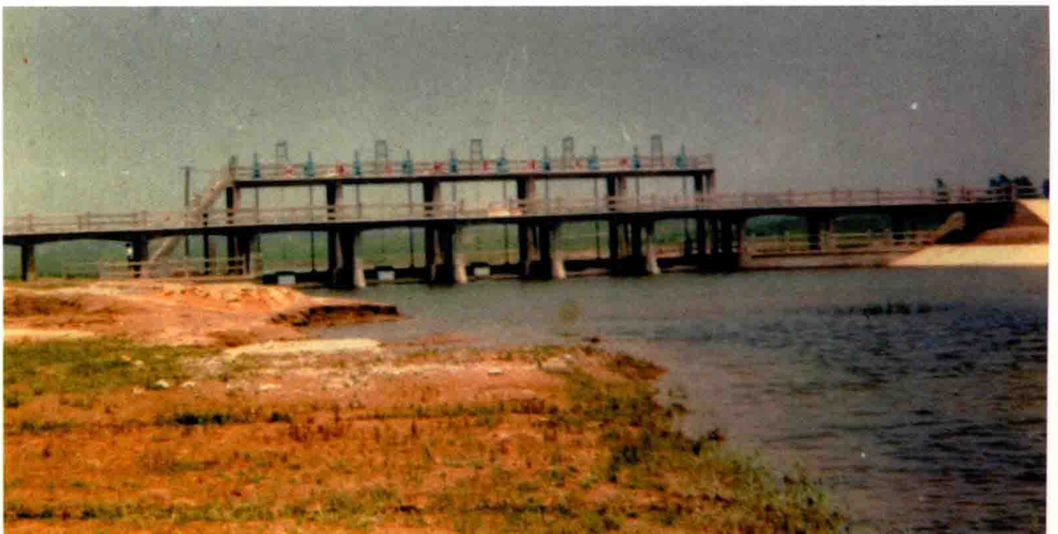
废黄河大兴漫水闸
