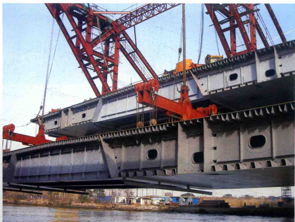
桥面吊机安装斜拉桥箱梁
