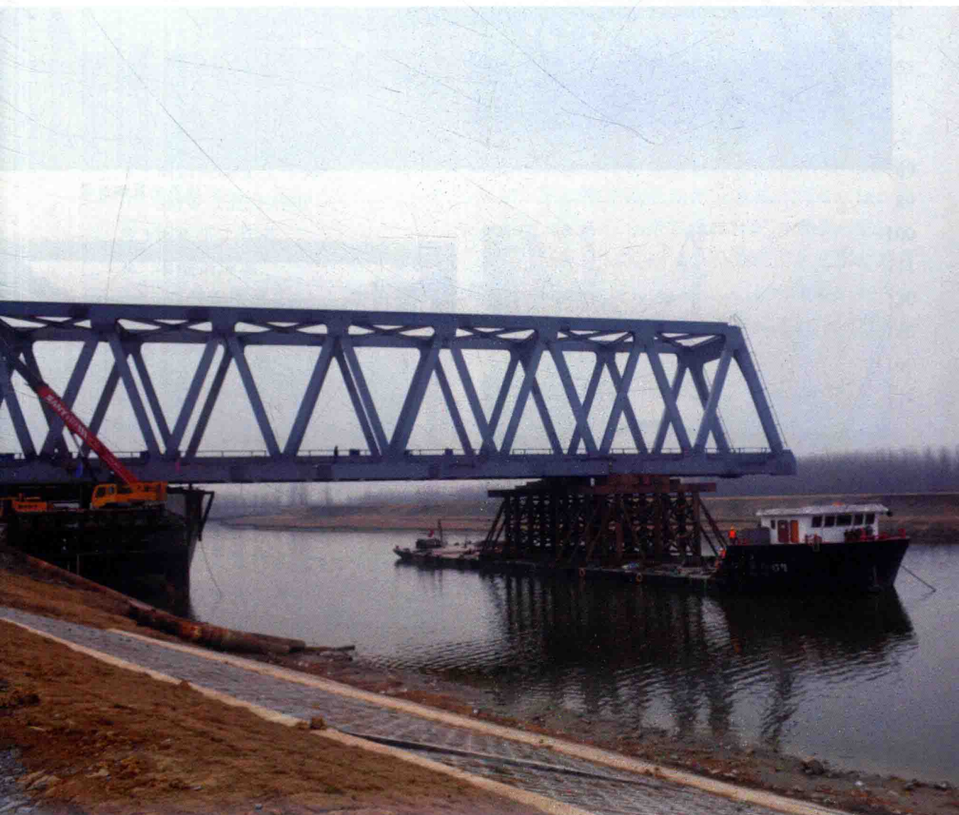
浮拖施工钢桁梁
