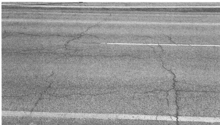
b. A Typical Non-load-Associated Cracking
