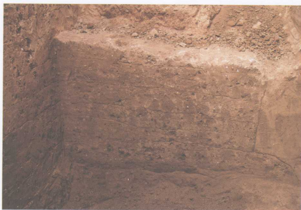
东壕沟 TG3 内夯土细部 Detail of the Rammed-earth Structure in Excavation Trench TG3 within the Eastern Moat
