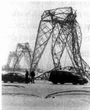
Fig.2 People look at a series of Hydro-Quebec high voltage towers near St-Bruno, Quebec, Canada, south of Montreal that collapsed after a severe ice storm hit southwest Quebec. The storm left more than 1.4 million households out of electricity.
