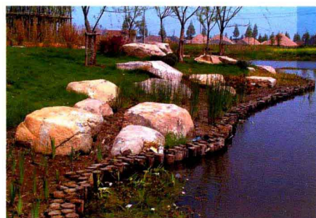
Notes on Engineering, Part Eleven 工程札记(之十一)——竹木桩驳岸
