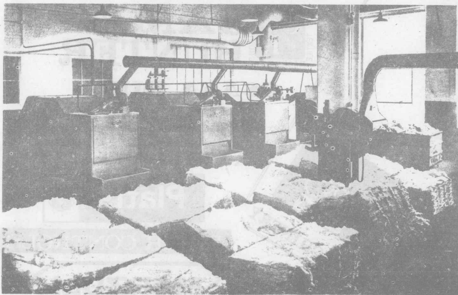
F-7 Feeders in the Opening Room of the Lyman Plant of Pacific Mills, at Lyman, S. C.
