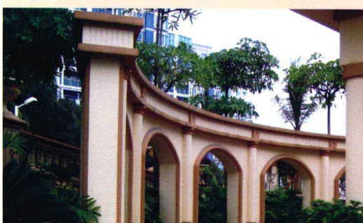
11-8 立柱、立廊 Upright Stanchion
