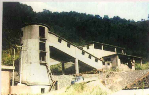
▲矿石输送走廊
