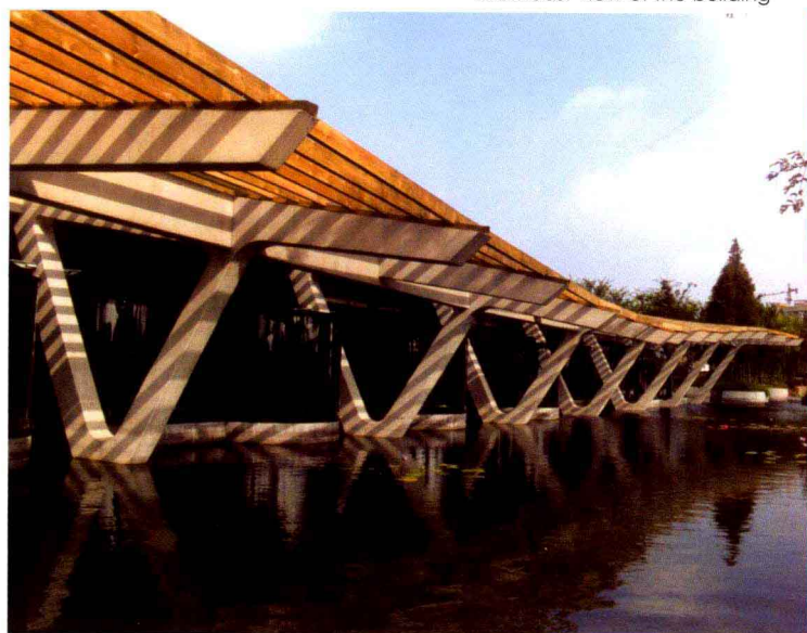
建筑东南角外观 Southeast view of the building
