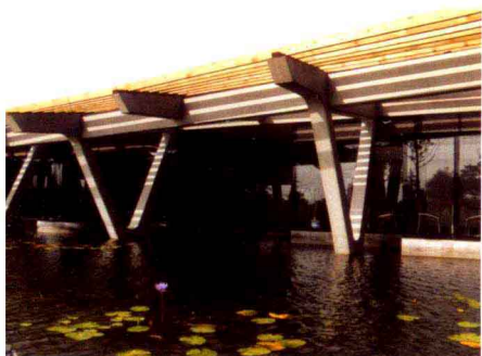
建筑东立面靠近主入口处局部 A part of the east elevation, behind which is the main entrance
