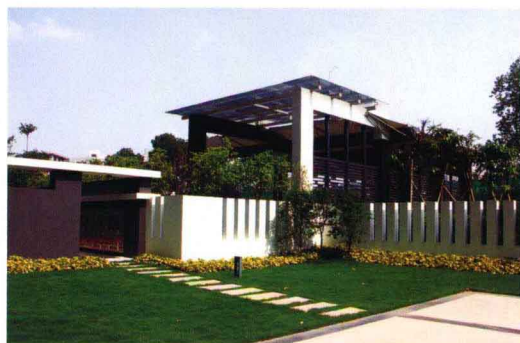
7-3 区域围栏、围墙 Fence & Wall
