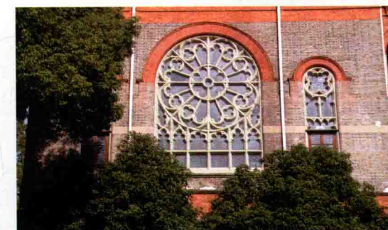
钟楼南面玫瑰窗 South Rose Window
