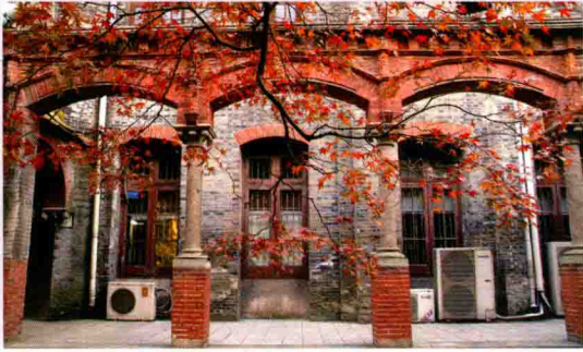
钟楼北面柱廊 North Arcade
