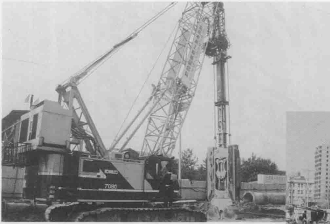
抓土机抓土开槽修筑连续墙
