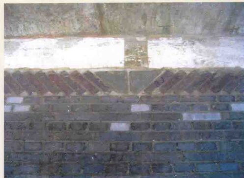
填充墙顶砼预制梯形块镶砌
