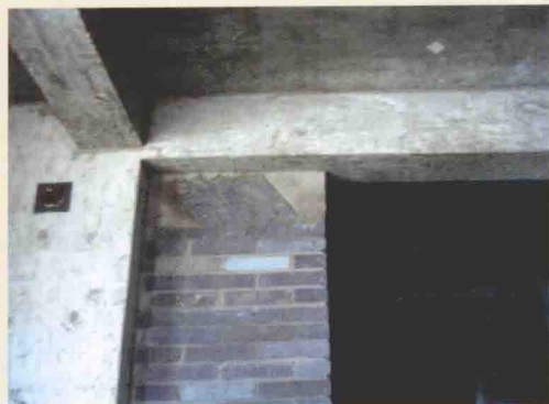
填充墙顶砼预制梯形块镶砌
