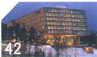
HEAD OFFICE FOR THE SWEDISH POST - THINK TANK 瑞典邮政总部大楼——智囊团
