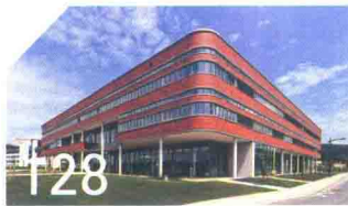
VILED A HEADQUARTERS 微力达总部大楼
