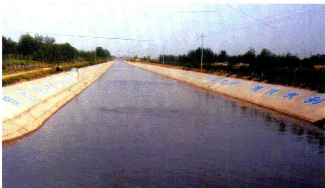
皂河灌区防渗干渠
