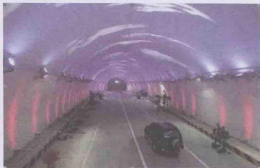
(a) 秦岭终南山隧道
