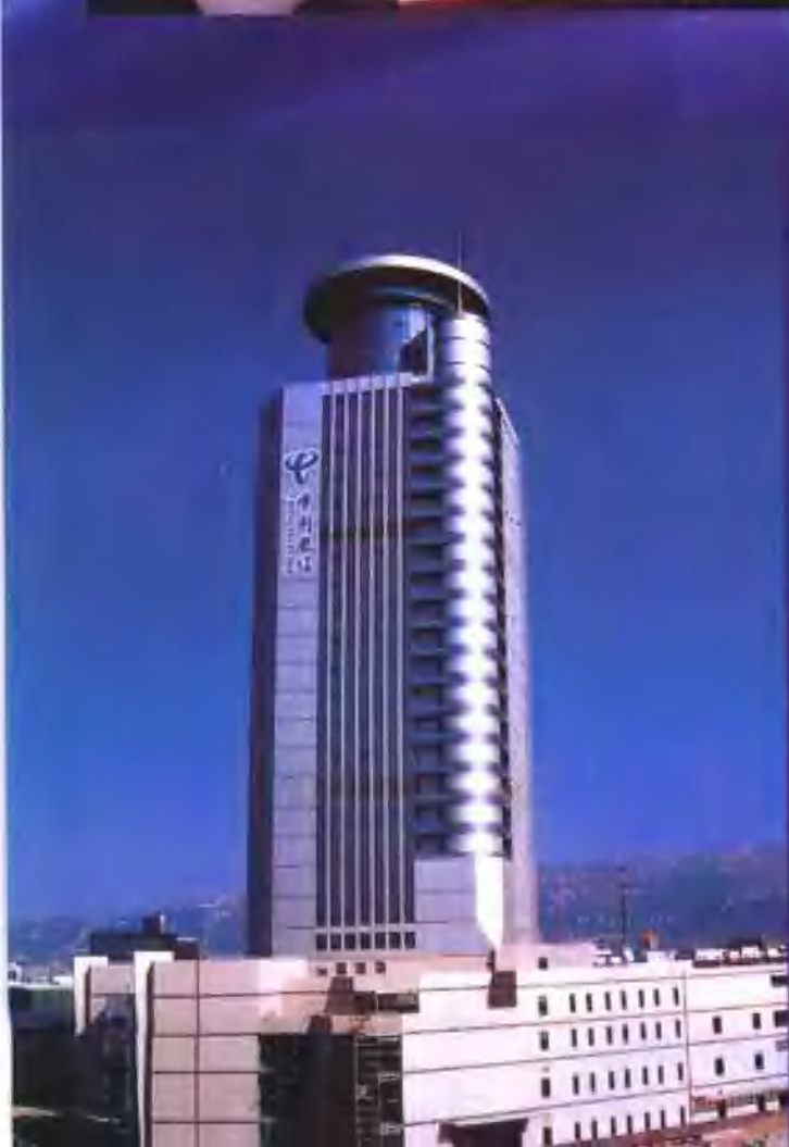
兰州第二长途电信枢纽 The second long-distance Telecom intersection of Lanzhou City
