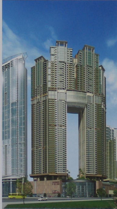
Residential Development Package 3 at MTRC Kowloon Station, Hong Kong
