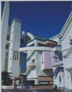
St Teresa's Church Annex 圣特利萨教堂副楼
