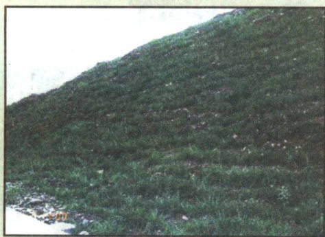
挖沟植草护坡
