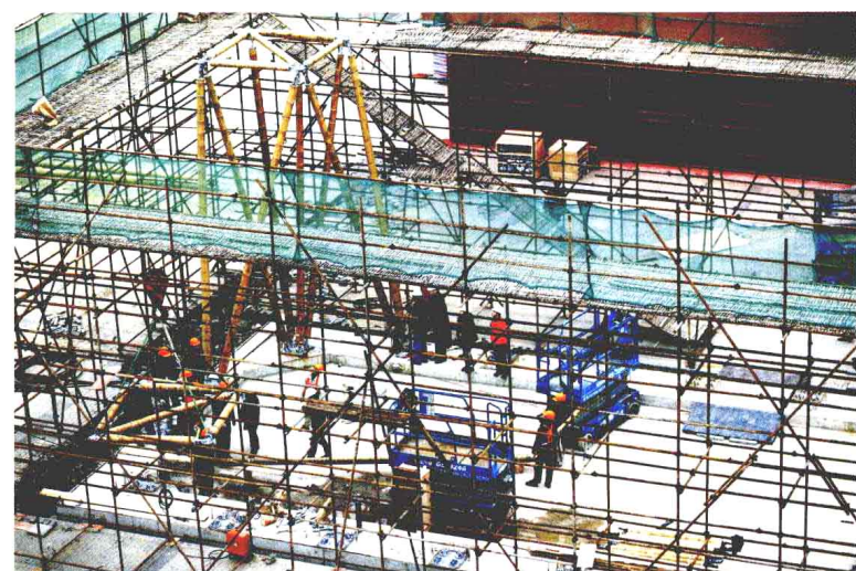
为德中同行之家展馆树立起的第一组竹支撑柱 Erecting the first bamboo supports for the German-Chinese House
