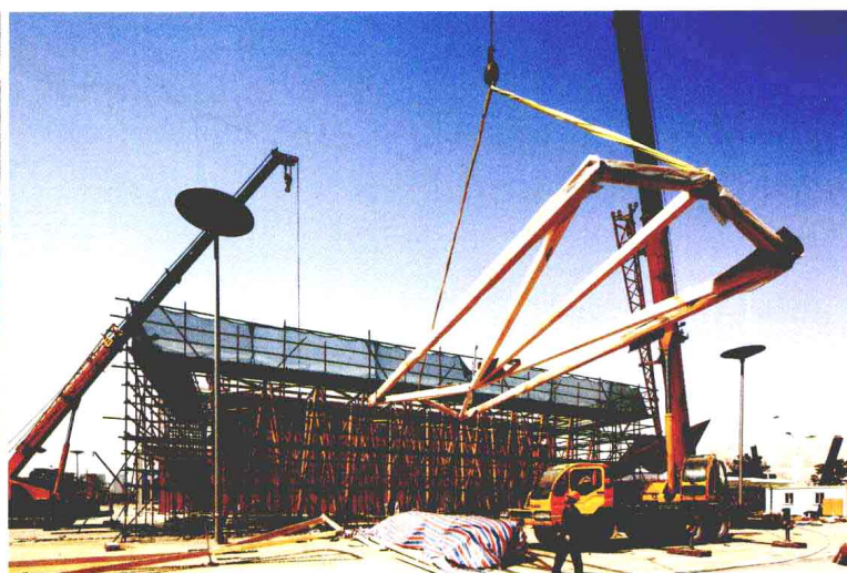
搭建过程——组装构成外立面的竹压板条 Assembling a facade element made of bamboo laminate
