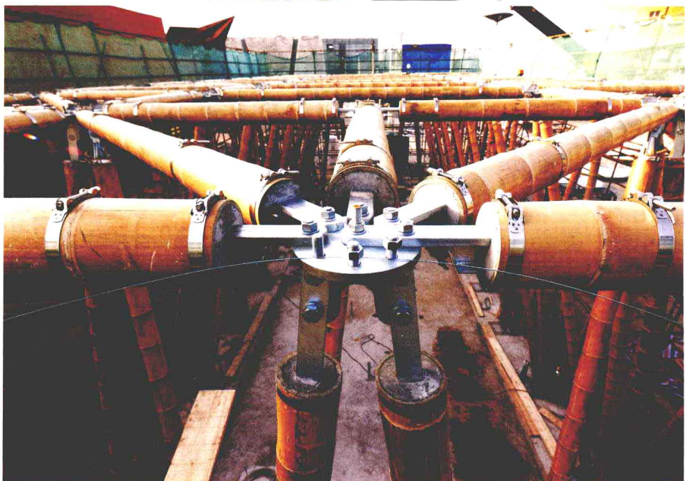
可调节接头集结点 Adjustable connection hubs for the bamboo rods
