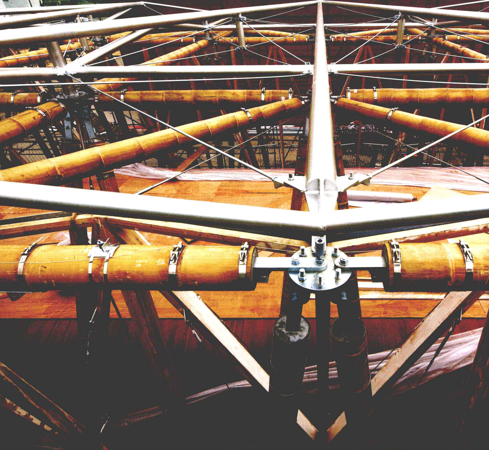
处于基础搭建阶段的顶部节点 Roof nodal points in the foundation during construction
