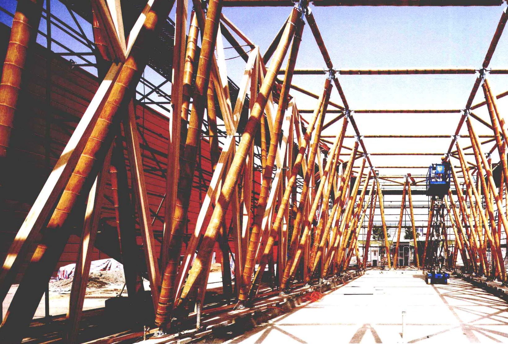
带螺栓的竹压板外立面框架 竹杆构成的V形主体结构 Bolt-on connection of the bamboo-laminate beam facade and V-shaped main structure made of bamboo rods
