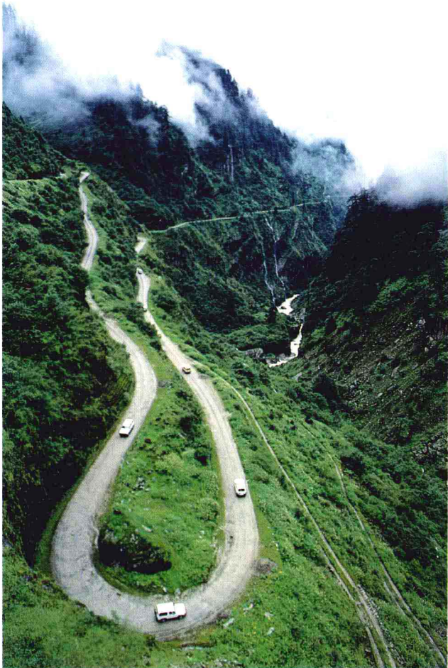
中尼盤山公路 The China-Nepal Highway with its twists and turns
