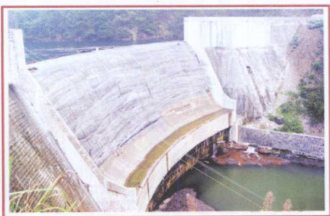
八舟电站大坝
