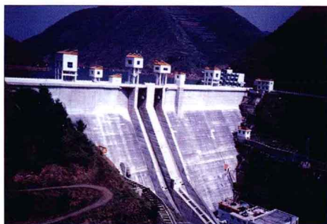
渔洞水库大坝
