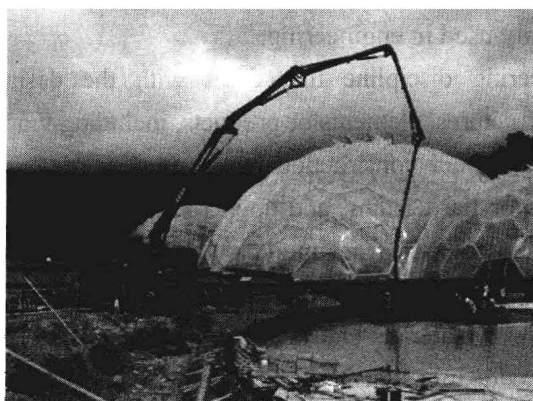
Fig.1-1 Pumping concrete construction
