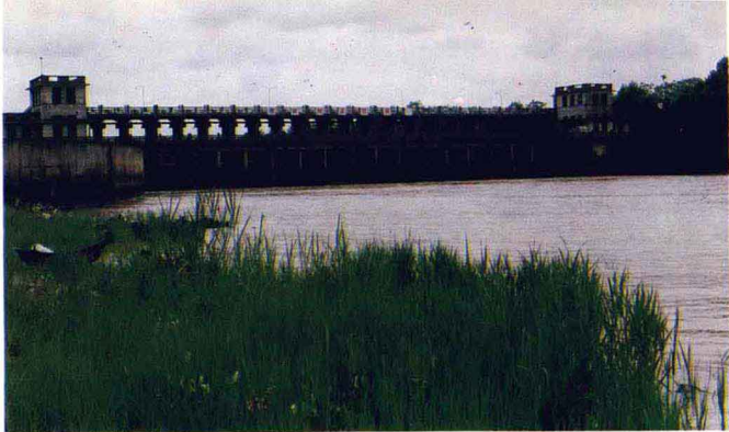
灌溉总渠腰闸
