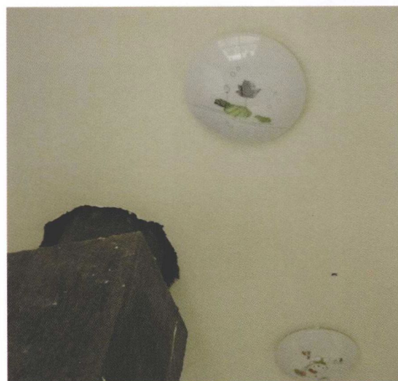
13 GNSS 观测墩与观测室软接触照片
