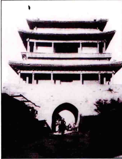
广安门旧城箭楼 The former gate tower of Guang'anmen
