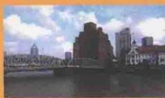
外白渡桥 Waibaidu Bridge
