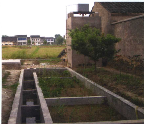
农户生活污水处理系统（生态过滤床—人工湿地池） Family sewage treatment by biological filter bed and wet- land, Jiangsu Province
