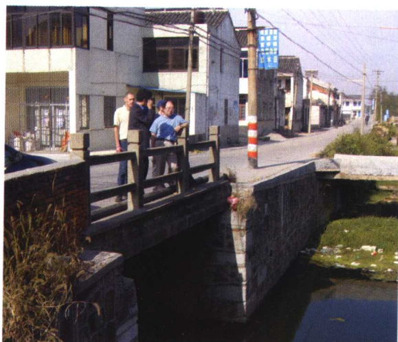
江苏宜兴农村生活污水排放引起的河道污染 Town river pollution caused by solid and liquid domestic waste in Yixing, Jiangsu Province
