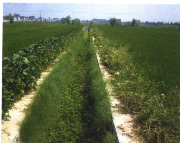
江苏宜兴农田面源污染治理的生态沟渠（种草和水生蔬菜）技术 Ecological ditch to control non-point pollution, Jiangsu Province
