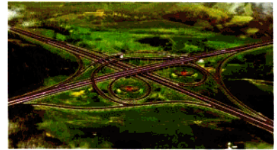
高速路立交 Interchange bridge of expressway
