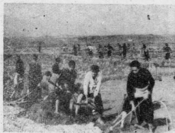
改良烂水田措施之三，挖塘泥
