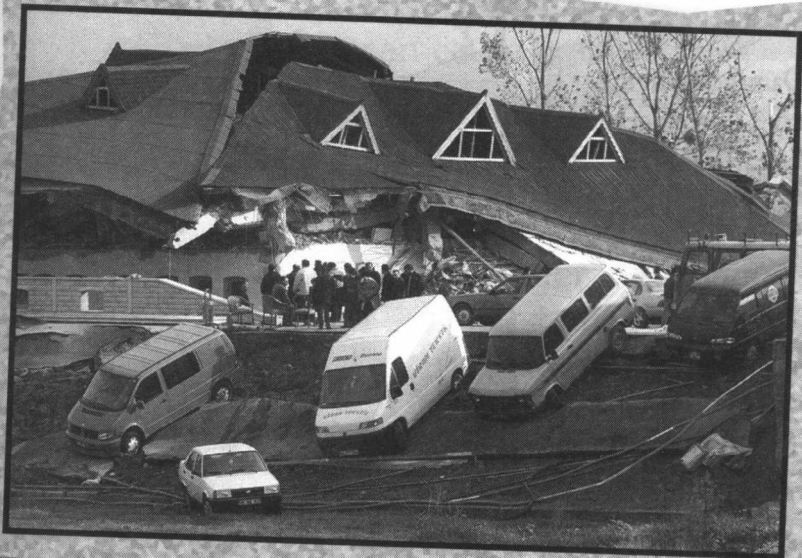
A parking lot and building are destroyed by an earthquake.
