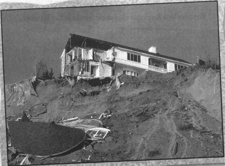
After an earthquake, a landslide caused more damage to this house.
