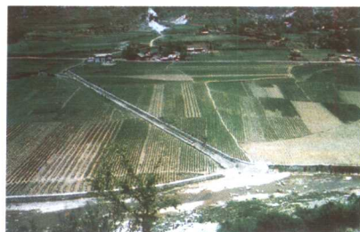
窝树坝子河堤
