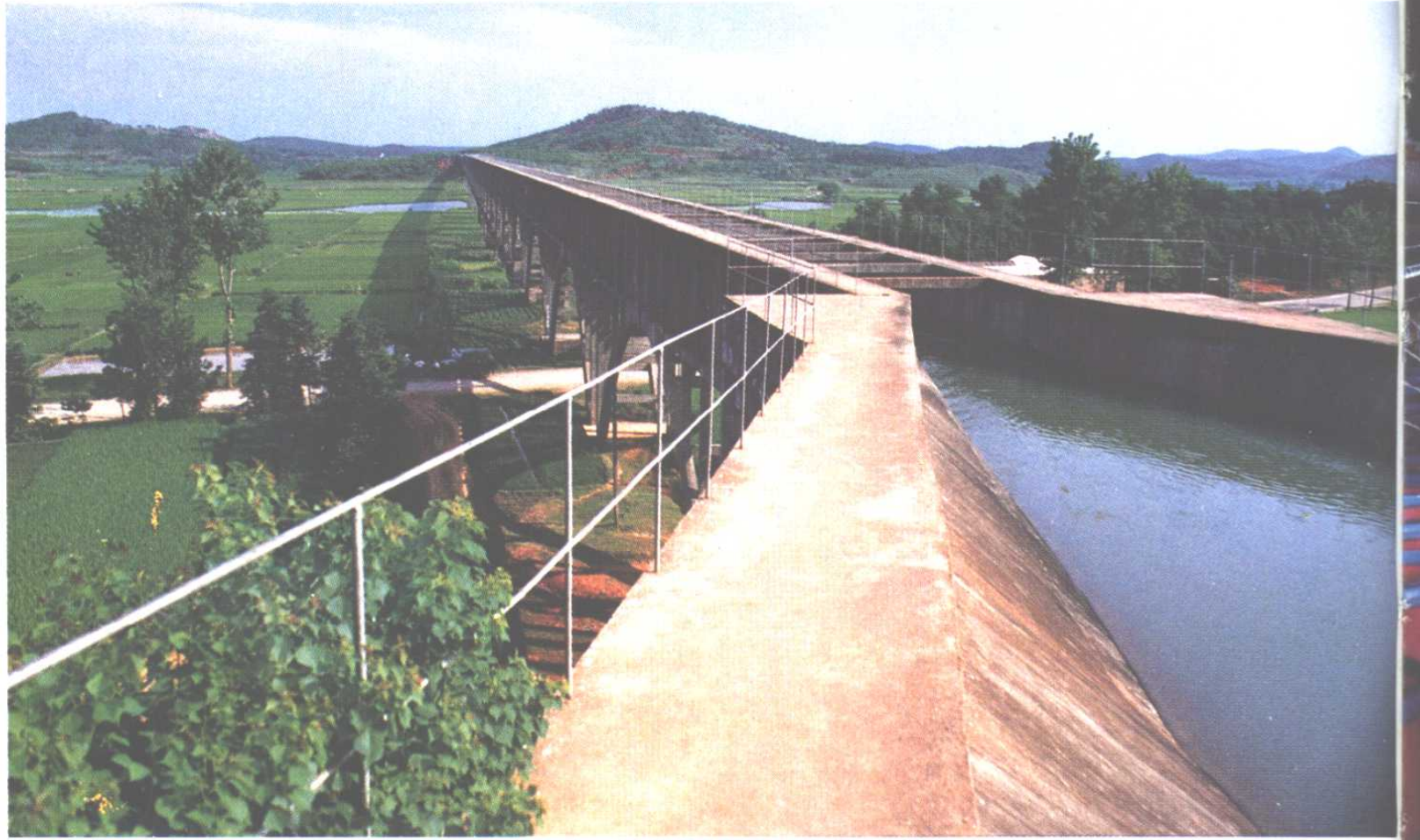
▶花凉亭灌区飞架的渡槽
