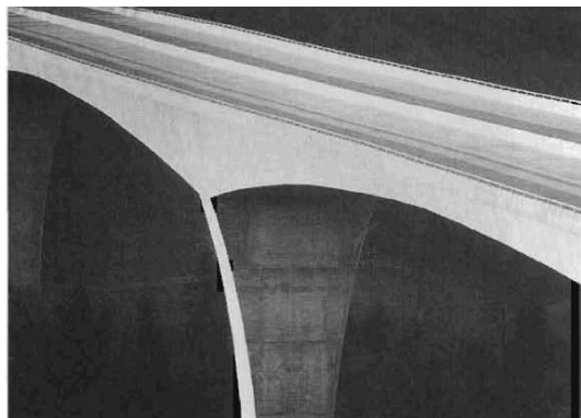
Fig. 1-9 Bennett Bay Centennial Bridge, Coeur d' Alene, Idaho, a four-span continuous concrete box girder structure of length 1730 ft (HNTB Corporation, Kansas City, Missouri).
