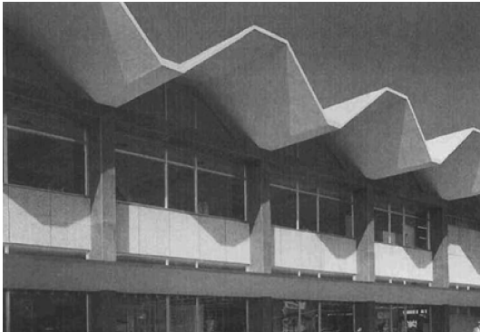
Fig. 1-5 Folded plate roof of 125 ft span, in addition to carrying ordinary roof loads, carries the second floor as well from a system of cable hangers; the ground floor is kept free of columns.
