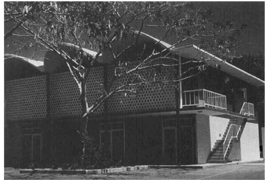
Fig. 1-6 Cylindrical shell roof providing column-free interior space.
