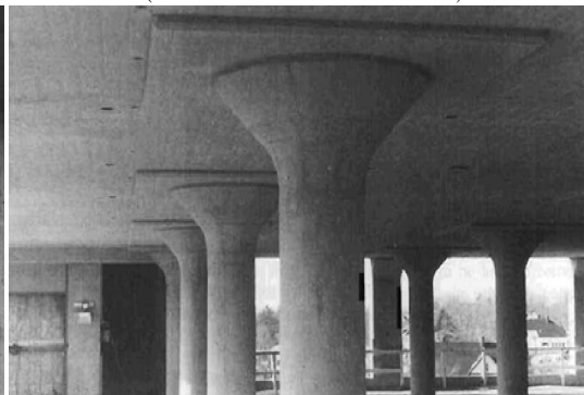
Fig. 1-4 Flat slab floor, without beams but with slab thickness increased at the columns and with flared column tops to provide for local stress concentration of forces.
