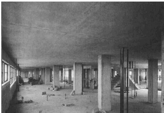
Fig. 1-3 Flat plate floor slab, carried directly by columns without beams or girders (Portland Cement Association).
