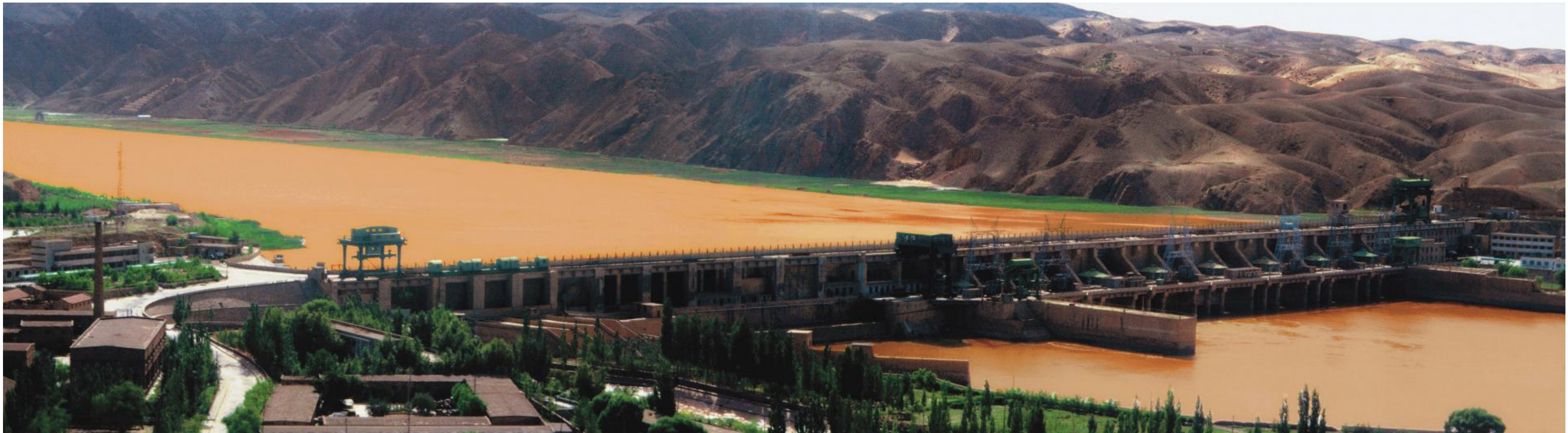
峡谷水库——青铜峡水利枢纽 The Reservoir in the Gorge – Hydrojunction of Qingtongxia
