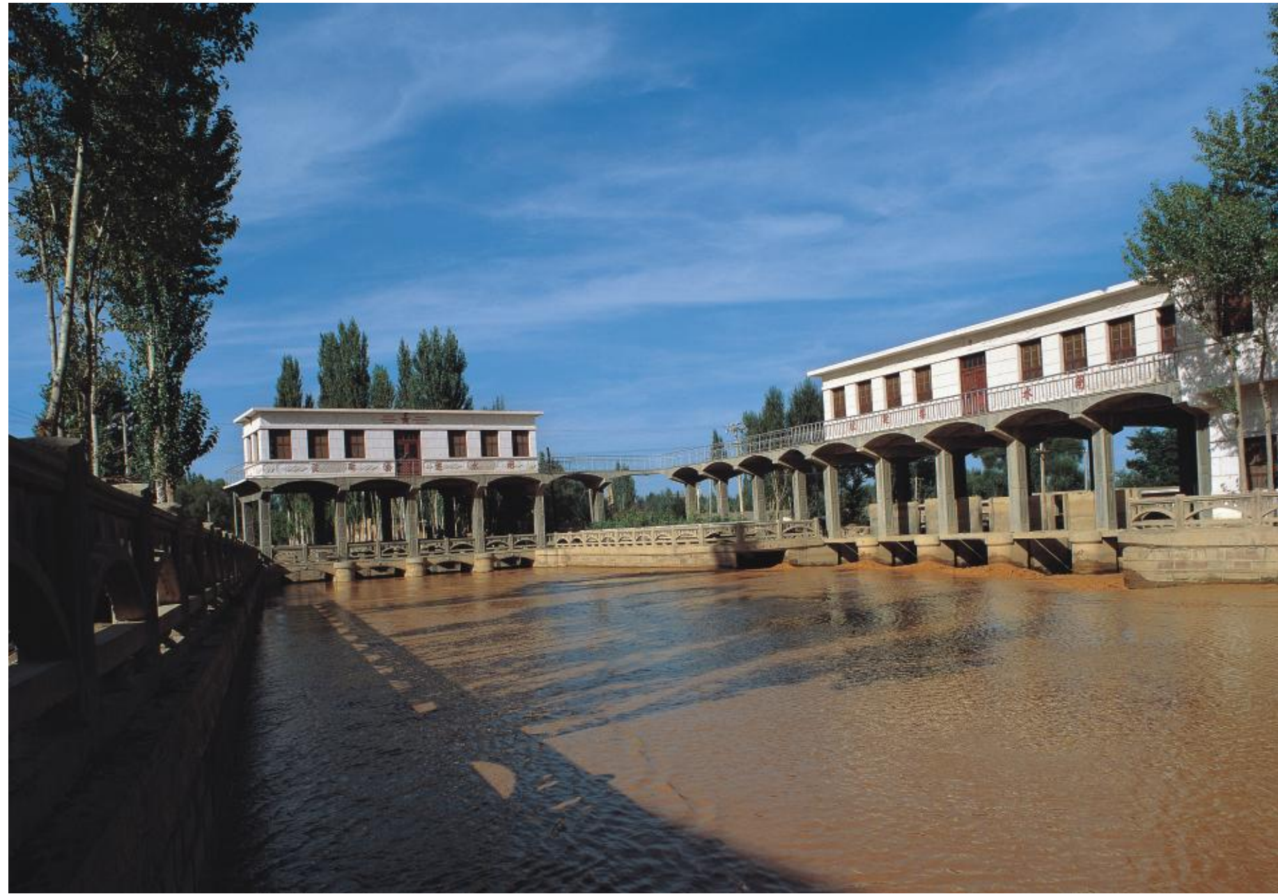
古渠：秦汉渠分水闸 The old Channel: the Diversion Sluice of Qin Channel and Han Channel
