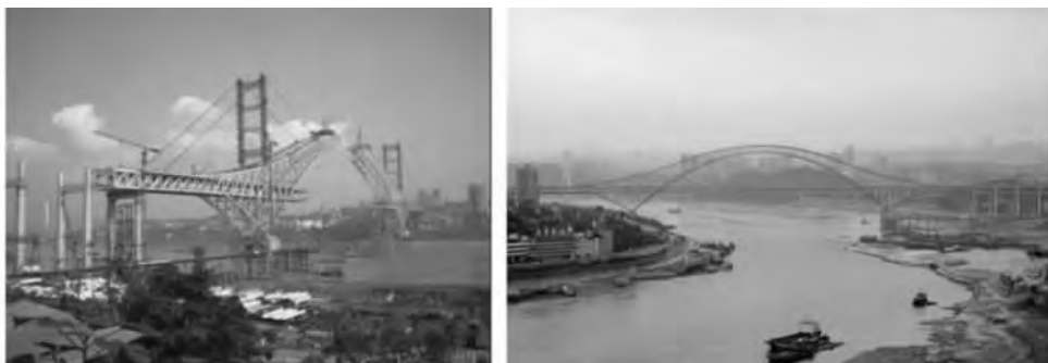
Fig. 7 Chaotianmen Bridge — During Construction and the Completed Bridge
