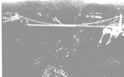
f)矮寨大桥(悬索桥)
