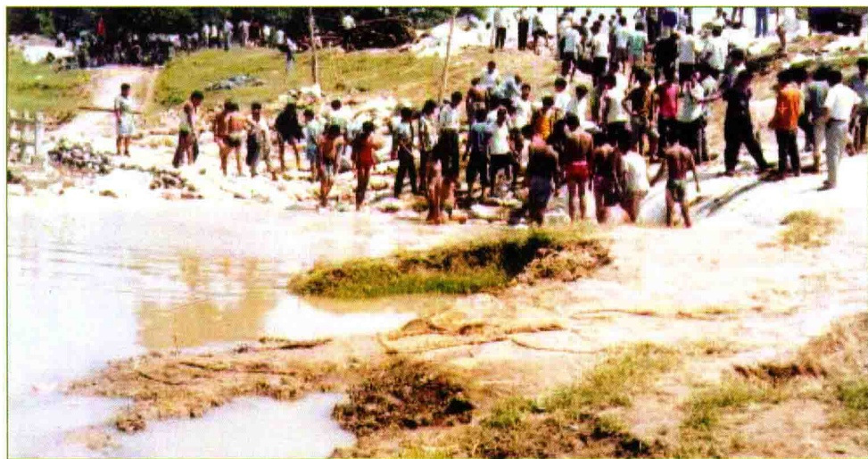
漳卫新河严务涵闸抢险加固
