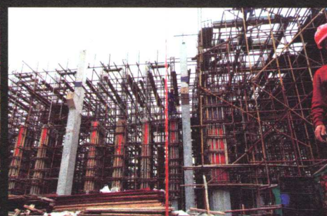
旧厂房混凝土立柱整体搬迁。 The concrete columns in former workshop were overall relocated.
