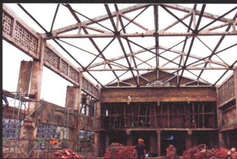
搅拌站原有框架结构得到了较为完整的保留。 The original framework of mixing plant was reserved completely.
