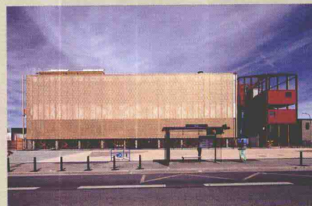
市郊学校TINO体育馆的南立面，外墙覆有装饰性的网状木板 south facade of gym, TINO, Inter-Municipal School, clad with decorative wood mesh panels
