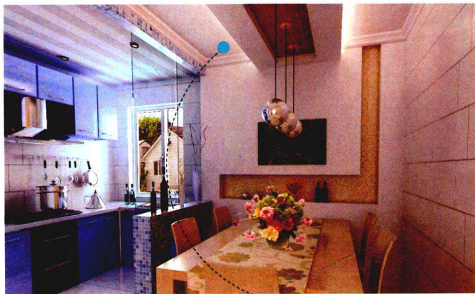
纸面石膏板+木板悬吊顶
