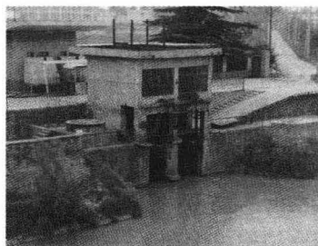
(a)原郑州花园口东大坝引黄闸
