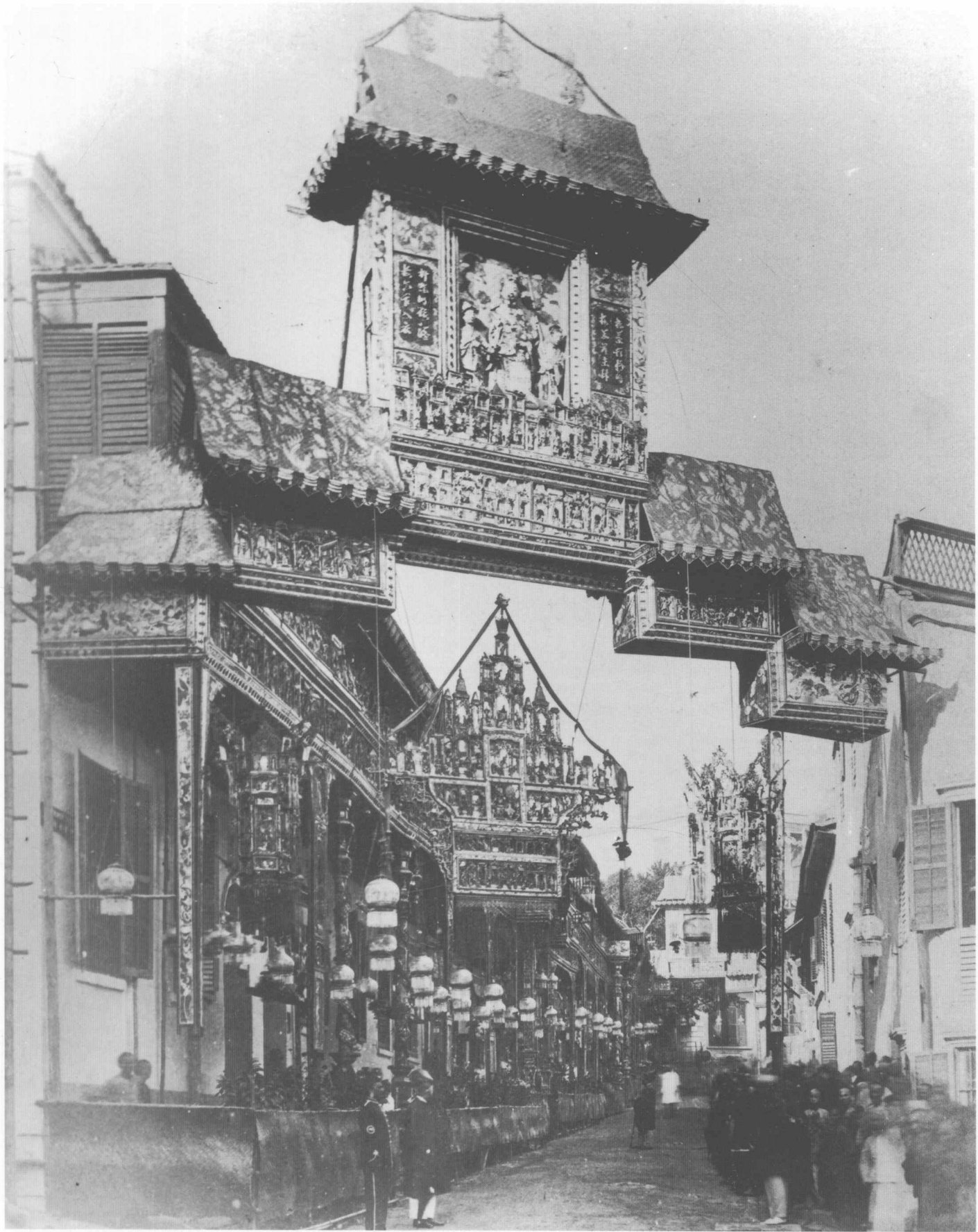
由閣麟街向西望擺花街，街上遍綴節日的裝飾，約攝於1880年。圖左為一黑底白字的路牌，“倫核士街”四字依稀可見。 Cochrane Street looking west towards Lyndhurst Terrace, c.1880. Festive decorations fill the streets. A street marker for Lyndhurst Terrace is visible on the left.
