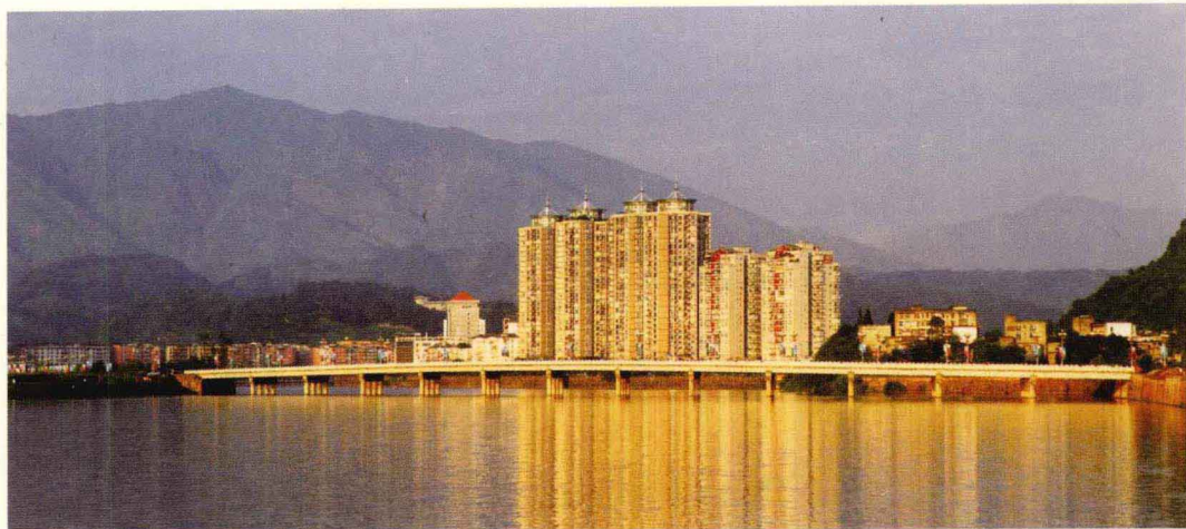
● 青衣江大桥 ● Qingyi River Bridge
