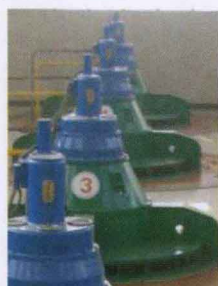
ZL 大型全调节立式轴流泵 Vertical Axial Flow Pump With Blades Pitch Adjustment
