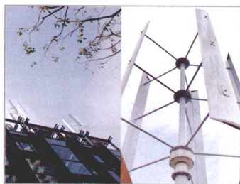
屋顶小型垂直轴风力发电机 Small Vertical-axis Wind Turbines on the Roof
