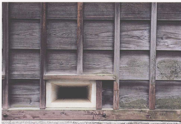
WA-10 木制框架结构，填入装有陶瓷通风口的弦切式厚杉木板 Timber-frame construction with infill of plain-sawn cedar planks with ceramic ventilation opening
