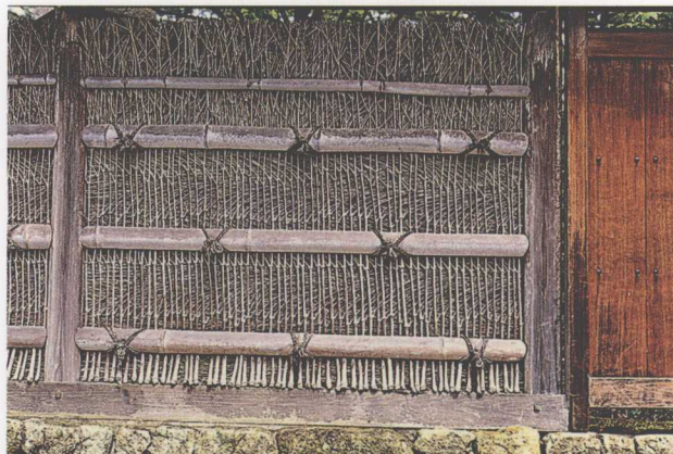
WA-12 编织的竹条系在竹子支柱和横杆上，花园栅栏 Woven bamboo twigs tied to bamboo post and rails, garden fence
