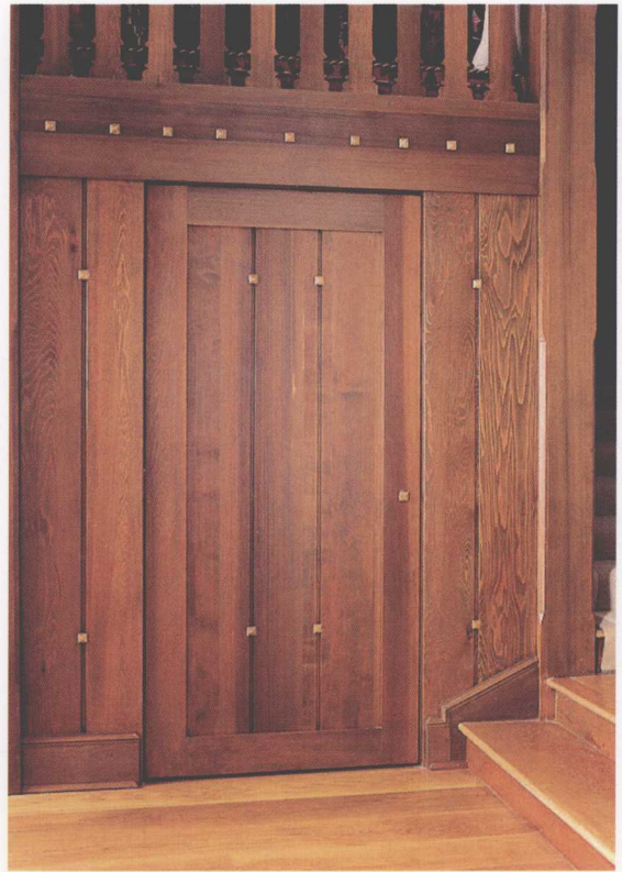
WA-19 框架式漆油杉木垂直镶板, 室内门厅 Framed oiled cedar vertical board paneling, interior hallway
