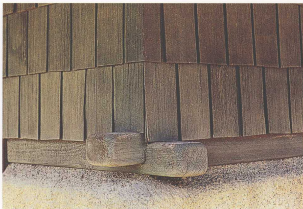
WA-9 方形木框架形成V字形切口拐角连接，喷漆杉木叠嵌在混凝土基座上 Notched corner joint of square timber frame with painted cedar shakes on concrete foundation
